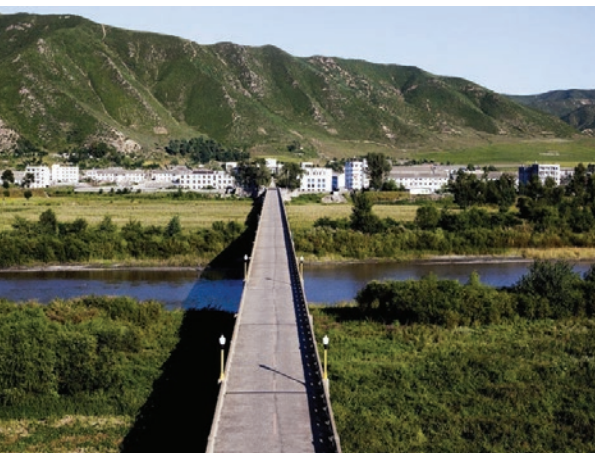
Bridge built in 1941 over the Tumen River, connecting North Korea with China.
